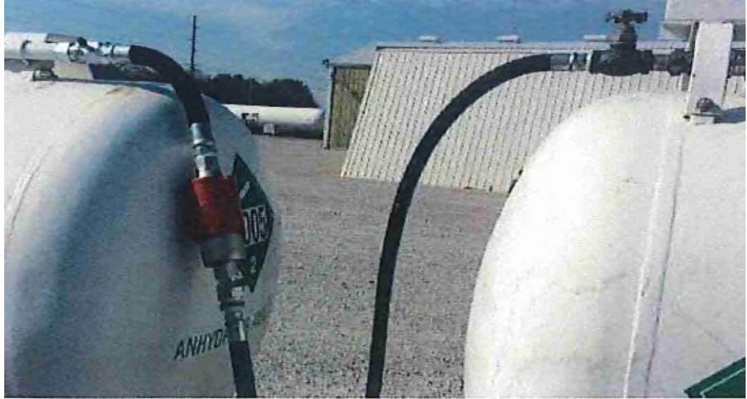
IB125 - Tandem Tank Installation
