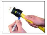
**7** Stab pipe completely into fitting entrance.
