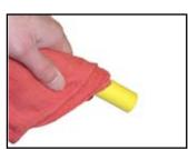
IMPORTANT: CHAMFER THE ID OF PIPE
