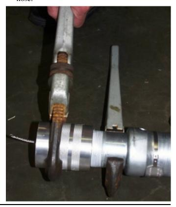
**9.** To eliminate the flat spots on the cable caused by the cap screws, use the hammer and chisel to cut the cable at a point just in front of the Sheath.
